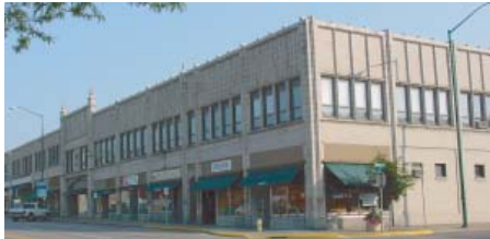
Mead Witter Building, West Grand Avenue (Recently purchased by G & J Properties)
